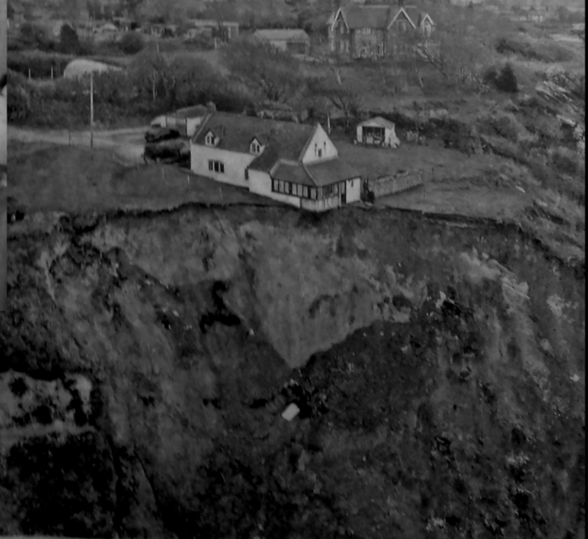
Cliff hanger A house has been left partly hanging over a cliff edge on the north Norfolk coast after a cliff fall destroyed. The owner of the three-bedroomed home at Cliff Farm in Trimmingham has been forced to ev
